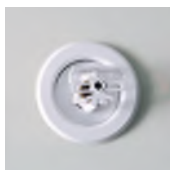
Sidewall Sprinkler
